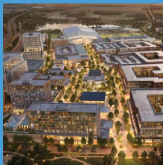
Bridgeland, TX Master Planned Community of the Year —National Association Home Builders
